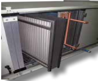
Fig 5: Eliminators installed on rails are removable for cleaning.
