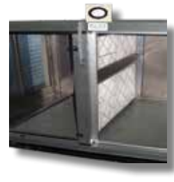
Fig 10: Pre Filter Section
